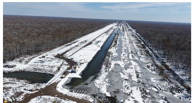
Levee Construction at WSLP-107
