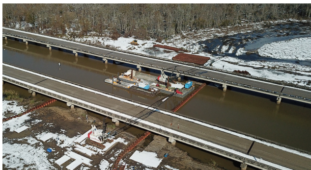
Levee and Floodwall Construction at WSLP-106
