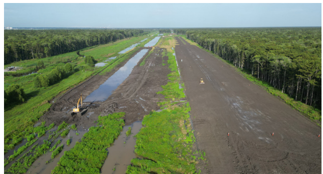
Levee Construction at WSLP-107
