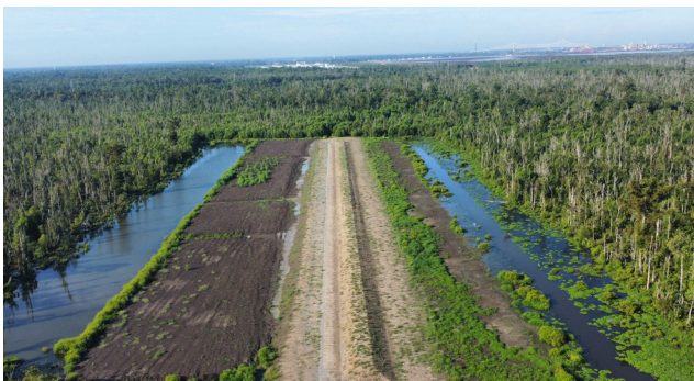
Levee Construction at WSLP-110
