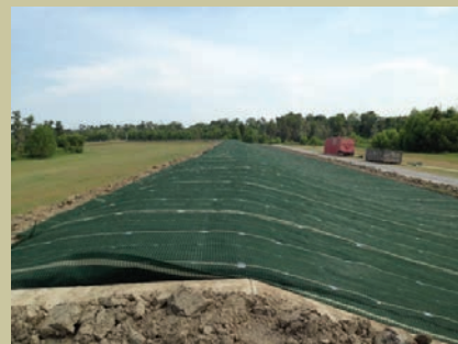
Armoring of Levee Reaches LPV-05.2a and LPV-05.2b
