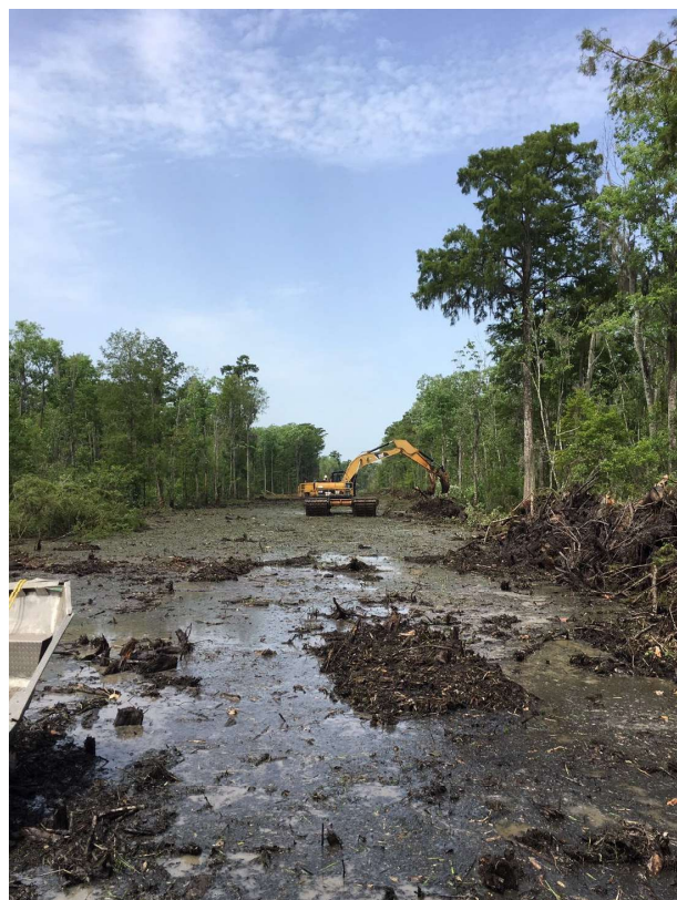
A 100' wide section of the West Shore Lake Pontchartrain levee footprint was cleared for surveying activities, including soil borings and other investigations
