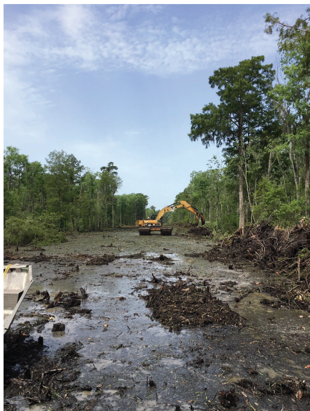
A 100' wide section of the West Shore Lake Pontchartrain levee footprint is being cleared for surveying activities, including soil borings and other investigations
