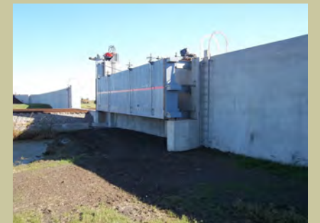
Illinois Central Railroad Swing Gate
